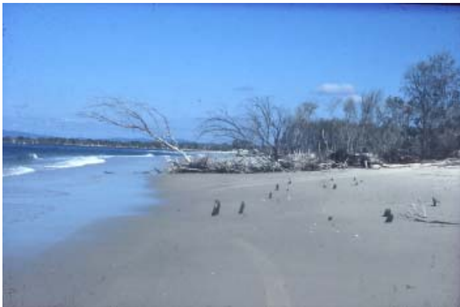
Figure B.10d. Jumpinpin downdrift bank 1997, looking west – evidence of erosion
